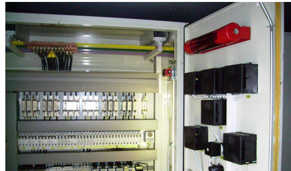
Electric Switch Board
